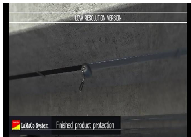
18] Fireproofing Protection on Build Strip PB
