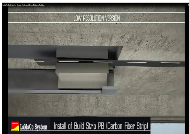
11] Install the Build Strip PB in Position
