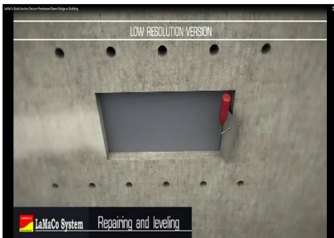
5] Patching to Leveling
