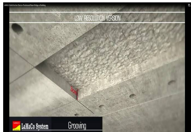
4] Hack Out or Grooving, Depth Set 30mm
