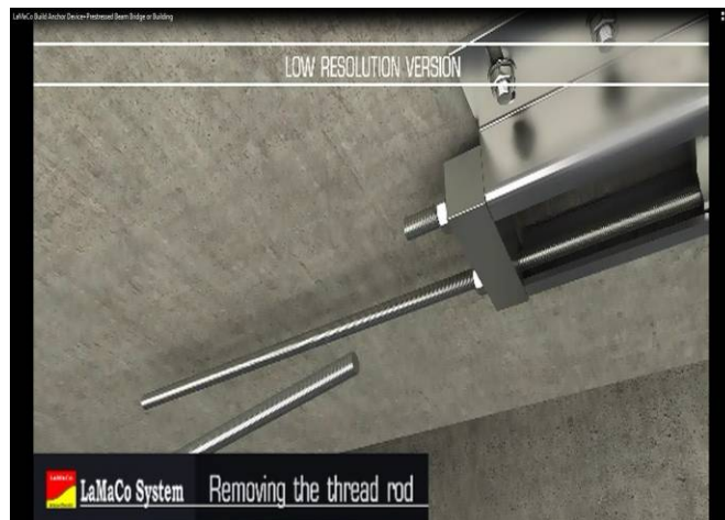
16] Once Finished, Remove the Thread Rod
